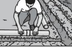
Test sub-surface for proper slope – should be minimum of 1%.
