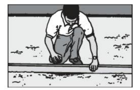
**c)** Mechanically prepare the area as required. For concrete, that does not have a broom finish around the area to be glued should be mechanically prepared (sandblasted or hand grinder) then cleaned to remove any dirt or dust. The same is for asphalt but a bond test should be done every time.
