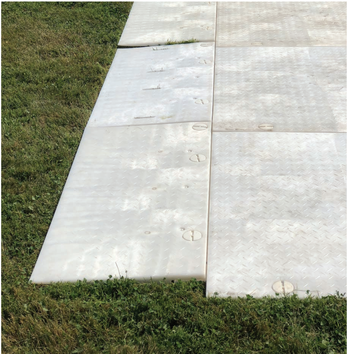
The first step is to lock male ramps in place along the entire length of the leading female edge of the panels.
