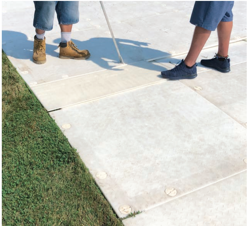
Install a row of female ramps over the male ramps, connecting them to the fresh row of panels.
