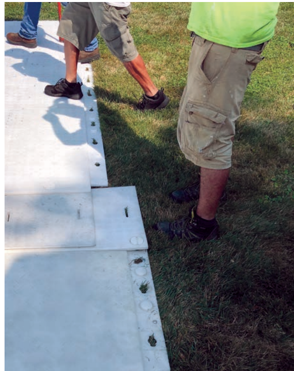
End of the HD/LD Build Joint.
