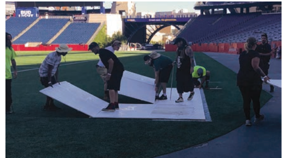
Lay the next pair of panels to extend the build in two directions.
