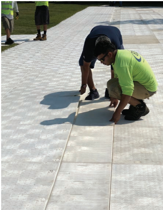
Complete the joint with a row of female ramps.
