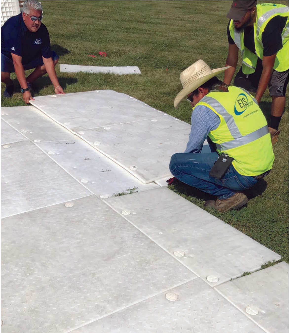
A fresh row of panels is placed along the leading edge of the male ramps.
