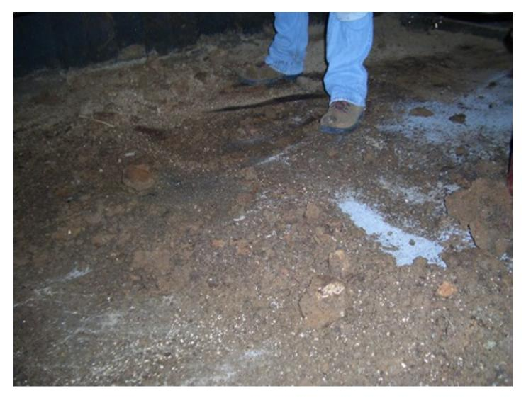
Pictured above is an uneven dirt sub-floor that we found in a customer's stall. I am sure you can see why it would not be ideal to lay your new stall flooring over this rough natural base.
