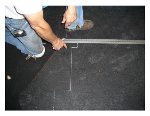
After you have your mat "sketched" out, it is time to begin cutting. Place your "T" square along the line to be cut. Put the blade of your utility knife alone the edge of the "T" square and using it as a guide, begin scoring the line to be cut with your knife. Score this line 3 to 5 times until you have cut over half way through the rubber.
