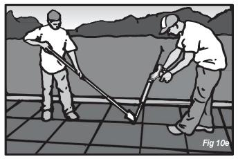
• Any excess adhesive should be left to fully cure prior to removal the following day. The excess adhesive can be quickly and neatly removed using a sharp razor knife.
