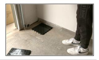
Keeping all additional tiles facing in the same direction, place tabs of new tiles over loops of already laid tiles and push down until they snap into place.
