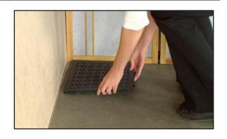
Keeping all additional tiles facing in the same direction, place tabs of new tiles over loops of already laid tiles and push down until they pop into place.
